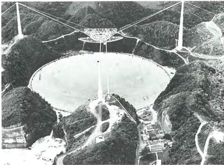
Left: The world's largest radio-radar telescope at Arecibo, Puerto Rico, is operated by Cornell. The spherical reflector has a diameter of 305 meters. The 600-ton feed support structure is suspended 150 meters above the reflector surface.
